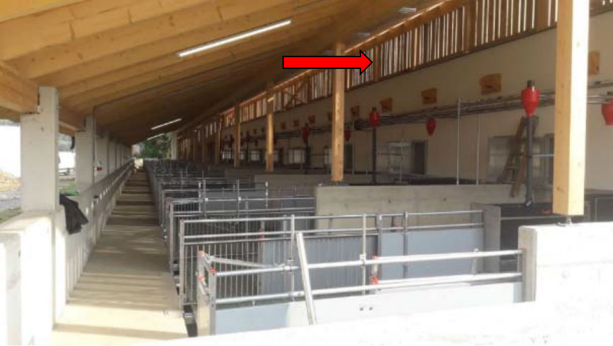
Abb. 4 Outdoor area with ventilation openings in the ridge area
