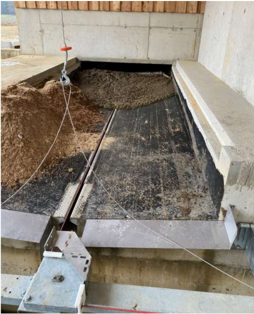
Abb. 9 Disposal (scrapers) with fecal urine separation
